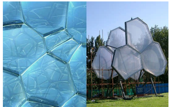
100,000 square meters of the Teflon-like translucent plastic ETFE
